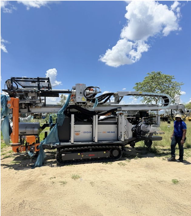
Figure 2: Sonic Drill Rig
